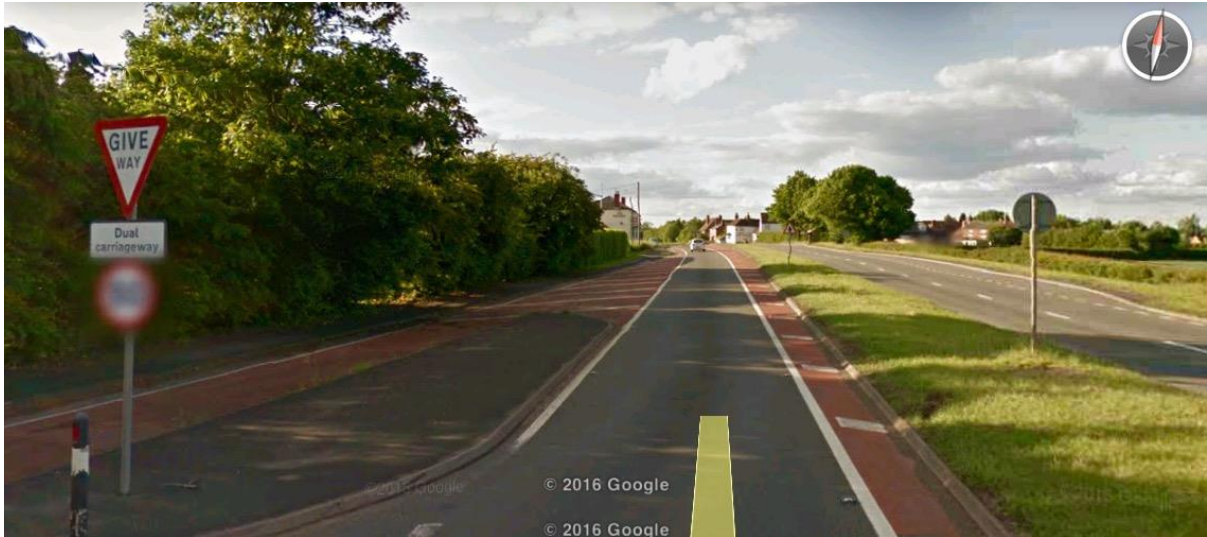
Photograph 6: The image shows a section of the A449 at Ombersley, Worcestershire (looking north). It has had its speed limit lowered and the road has been reduced in size from two lanes to one by Worcestershire County Council.
